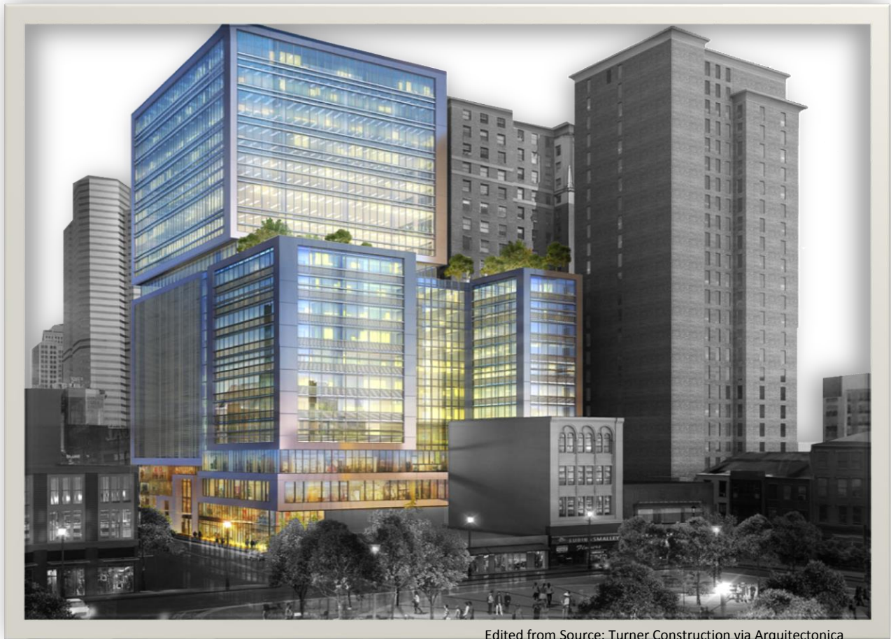
Edited from Source: Turner Construction via Architectonica
