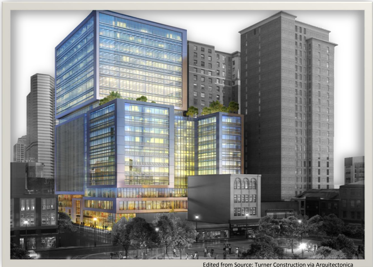
Edited from Source: Turner Construction via Architectonica
